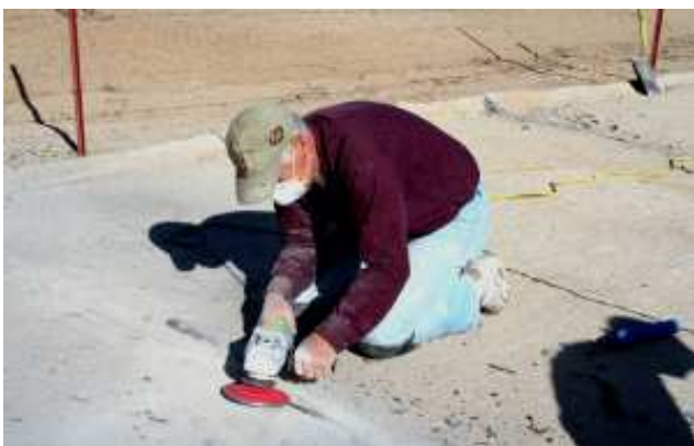
Below— Treasurer Phil Garro dons a dust mask and grinds old asphalt off the cracks in the rain apron. All this older patch material must be removed before the cracks can be filled with new cement and coated with Merlex sealer.
