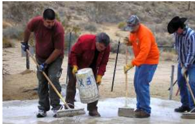
Below— Our hardy weekend work crew brooms Merlex waterproof stucco on finished rain apron on A16. This prevents rain water soaking into the concrete. All the rain that lands on the apron goes into the underground water tank.
